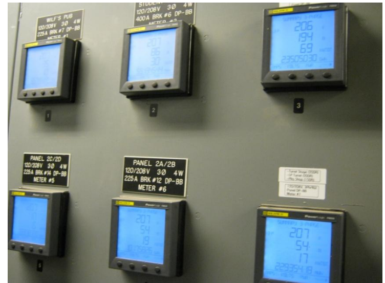
Electrical submeters
